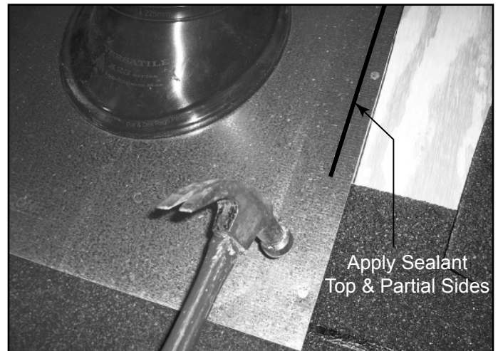
Figure 10.21 Slide Flashing Down, Secure & Apply Sealant
